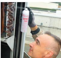
I use iBIOTEC DETECT 1000 for finding the exact location of refrigerant leaks. Electronic detectors give only a basic overall localization of leaks. The advantage of IBIOTEC DETECT 1000 is that the pressure remains constant, even in a low temperature environments. The leak detector I used previously didn't pump well when it was cold and produced very few bubbles.
